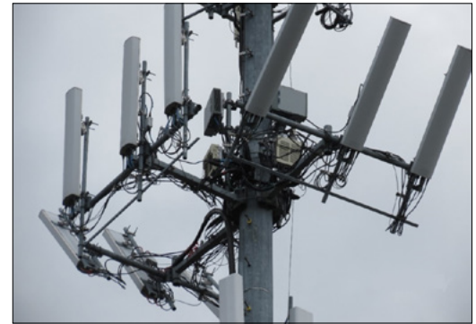
Figure 9 – T-Arm Mount Face Rotation
