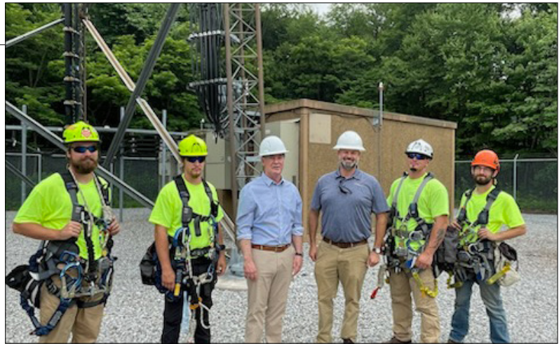
Congressman Joyce joined Christopher Mika and the Novotech Construction, Inc. crew at a tour site.
